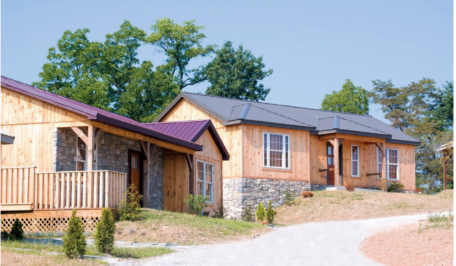
Structures at The Lodges at Gettysburg, a 62-acre private retreat, are shown. The Lodges has incorporated green technology at the property in the form of an underground, vertical closed loop geothermal system.
